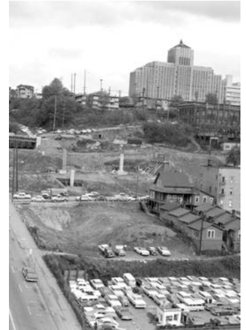
U.S. Interstate Highway construction in Seattle, Washington, in 1963.
